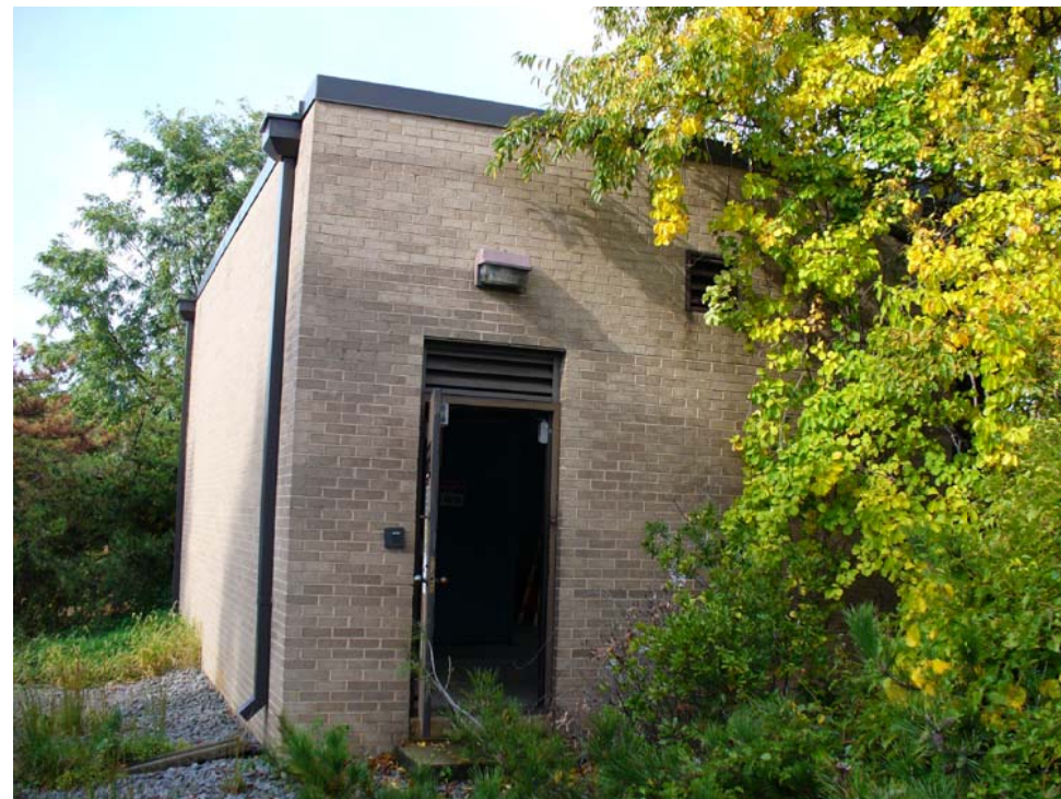
TIE BREAKER ACCESS
